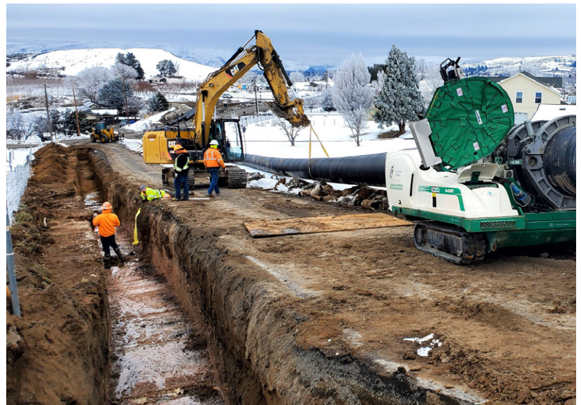
33" pipe being installed - No. 3 Lateral near 2.8 mile, Tibbling Rd.
