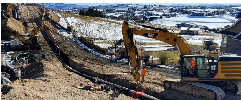
36" pipe being installed - No. 3 Lateral near 2 mile, Heather Heights Drive area
