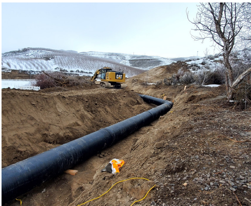
36" pipe being installed - No. 3 Lateral near 1.6 mile, Heather Heights Drive area
